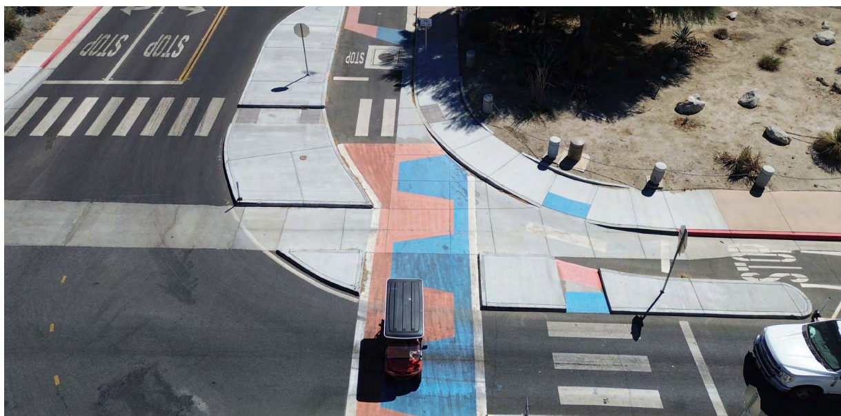
CV Link with crosswalks and protected intersection at El Cielo Road and Mesquite Avenue in Palm Springs
