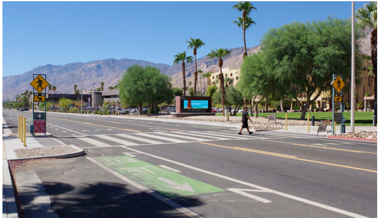
High-visibility pedestrian crossing and bike lane at the Palm Springs Convention Center
