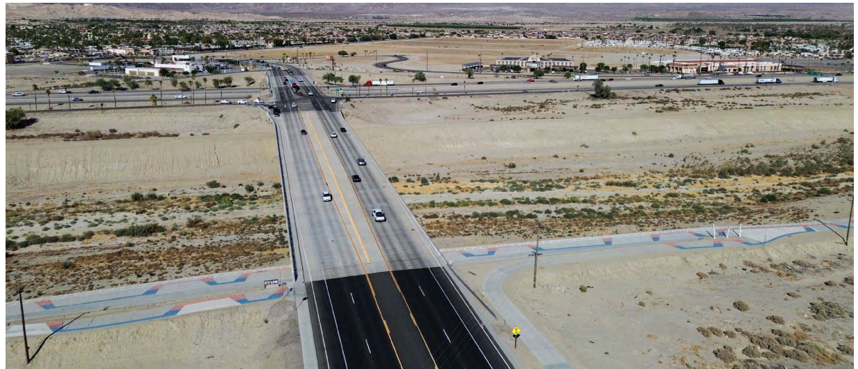
Golf Center Parkway, crossing Interstate 10 and Whitewater River (CV Link in foreground)
